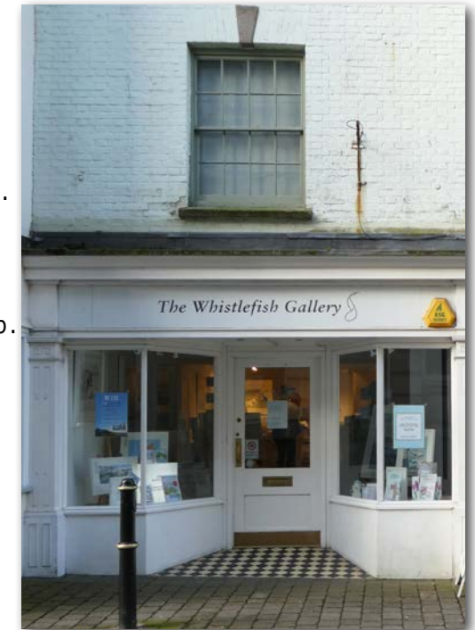
This shopfront in Falmouth has been created with a ramped, tiled threshold. The recess is splayed to improve access and the door is wide.
