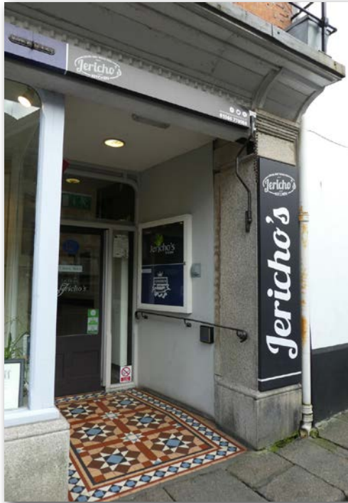
Jericho's at Liberty's in Launceston has an automatic push pad, an assistive handrail on the ramped threshold, wide door access and lift to the first floor restaurant.
