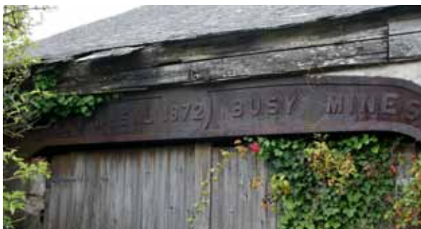
Above: Cast iron door lintel at Wheal Busy near Chacewater
